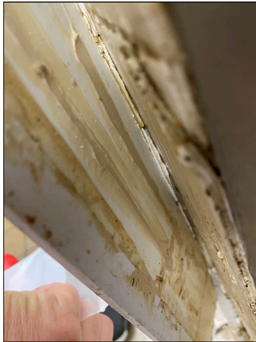
4 - HA-04: Non-ACM FRP mastic
