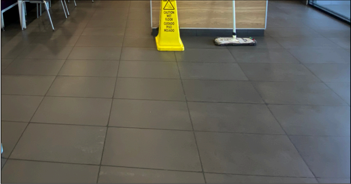
5 - HA-05: Non-ACM gray-black grout in FOH
