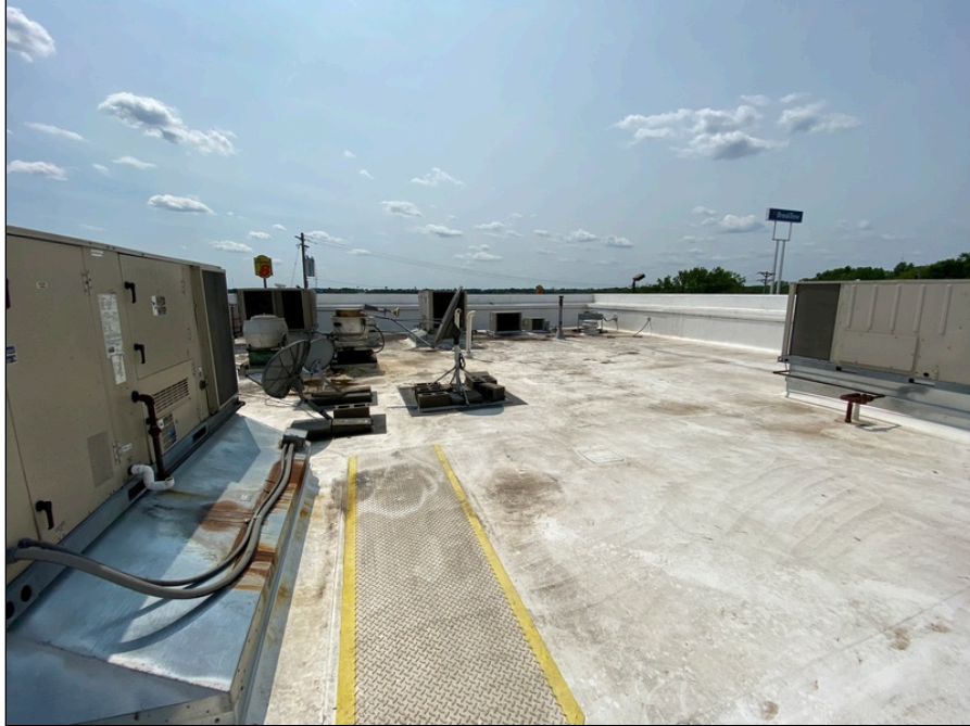
13 - HA-13: Non-ACM membrane roofing system (may be overlaying an inaccessible roofing layer)
