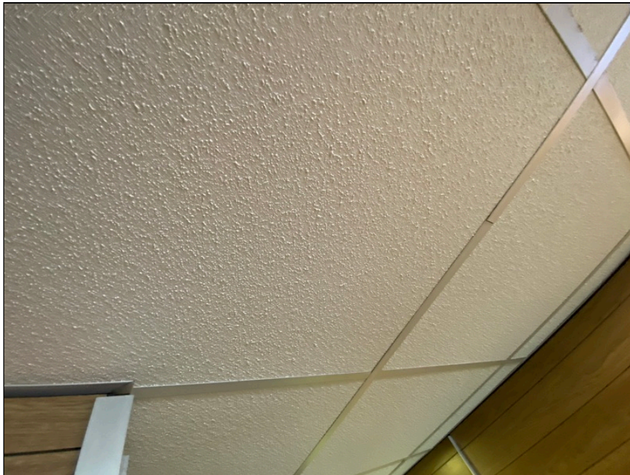
2 - HA-02: Non-ACM 2-ft by 2-ft textured ceiling tiles
