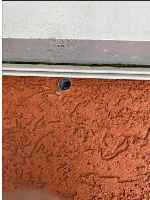
9 - HA-09: Non-ACM EIFS exterior building finish
