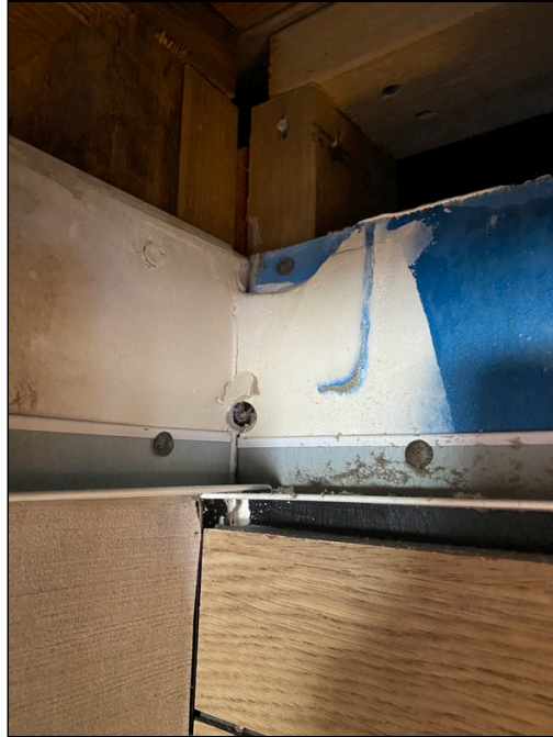
1 - HA-01: Non-ACM drywall and joint compound
