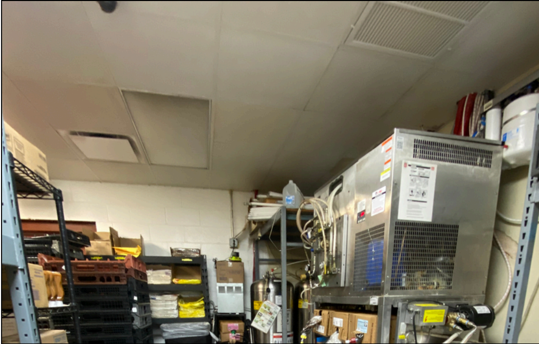
3 - HA-03: Non-ACM 2-ft by 4-ft fire resistant ceiling tile
